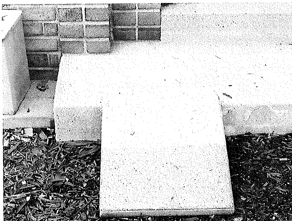
Above: Photo of sample of concrete to be employed. Sample is propped against concrete stoop, showing top half of sample unsealed & bottom half coated with sealer.
