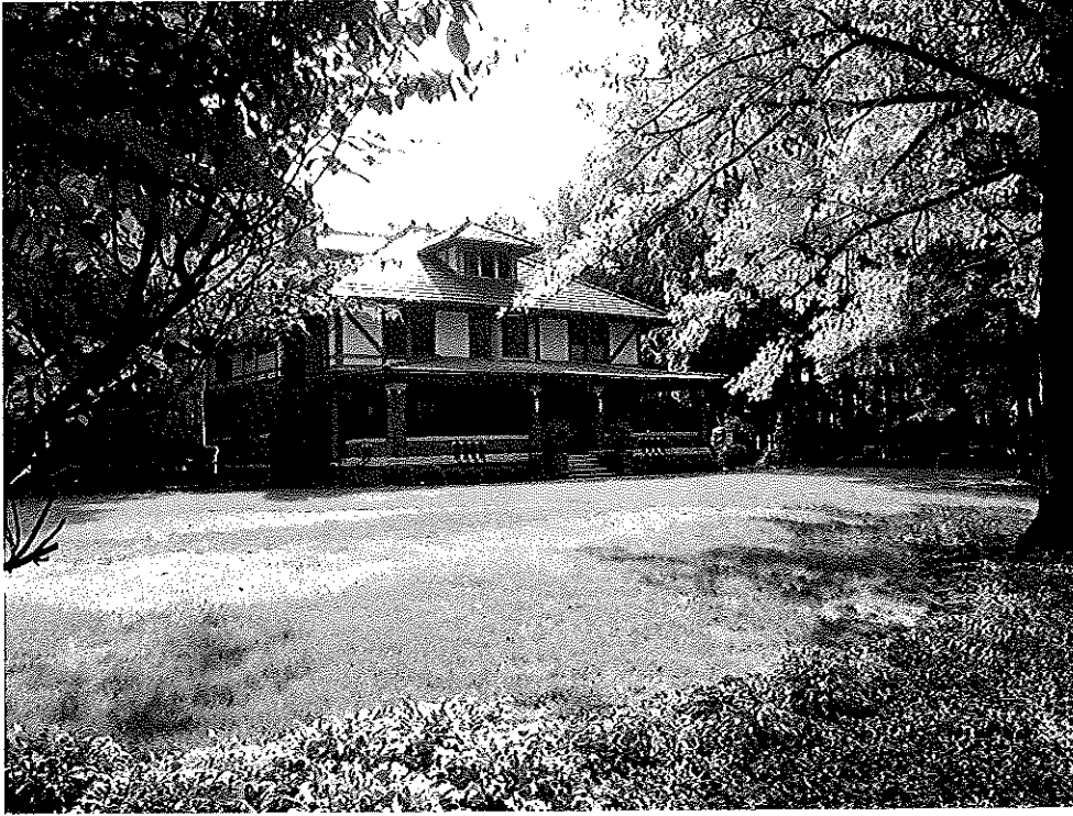
Rear of home where construction is to be done
